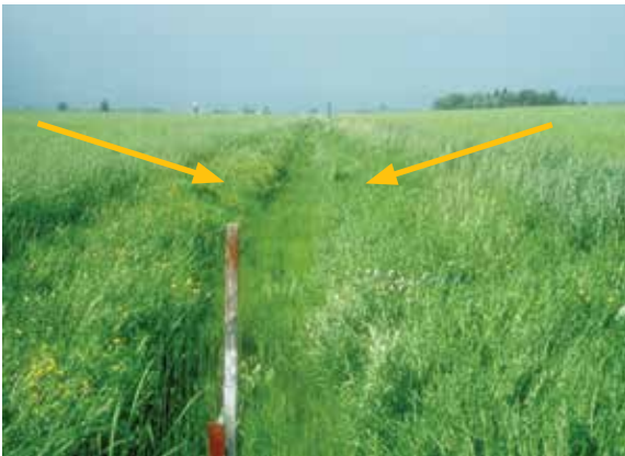
Figure 17.18. Surface drainage on clay soils in Ontario, Canada. Excess water travels over the surface to a grass waterway.
