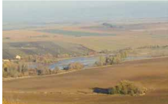
Figure 14.10. Top: A sediment control basin in a Central European landscape where conventional tillage is widely used. Bottom: Sediment regularly fills the basin and needs to be dredged.
