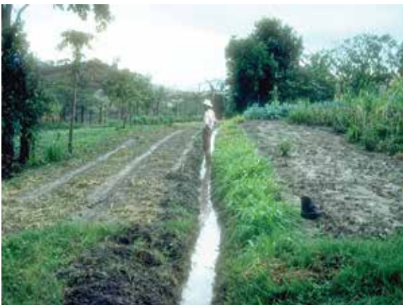
Figure 14.7. Hillside ditch in Central America channeling runoff water to a waterway on the side of the slope (not visible). A narrow filter strip is located on the upslope edge to remove sediment.
